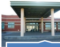
Dawson Creek and District Hospital
